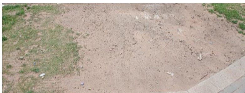
Example illegal driveway crossing
